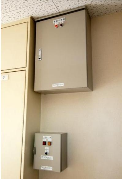
Two electrical control panels are mounted on a light-colored wall. The upper panel is larger and labeled '自動電源切替盤' (Automatic Power Switching Panel). The lower panel is smaller and labeled '自立運転スイッチ盤' (Independent Operation Switch Panel). Both panels have various switches and indicators. | <p>(上)自動電源切替盤<br/>(下)自立運転スイッチ盤</p>              |
